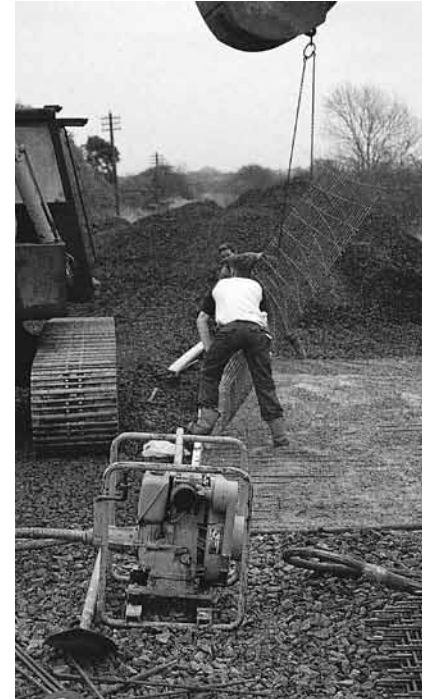
Reinforcing roof of Sett
