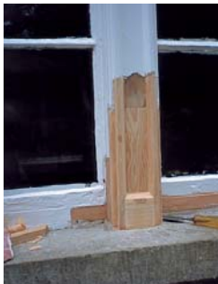
Degraded parts of a wooden window can be removed and replaced for a fraction of the cost of a replacement PVC- u window
