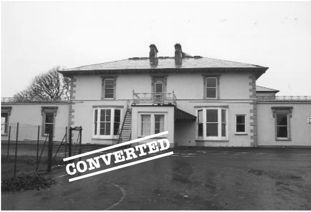
Former Special Care School, Killadeas
