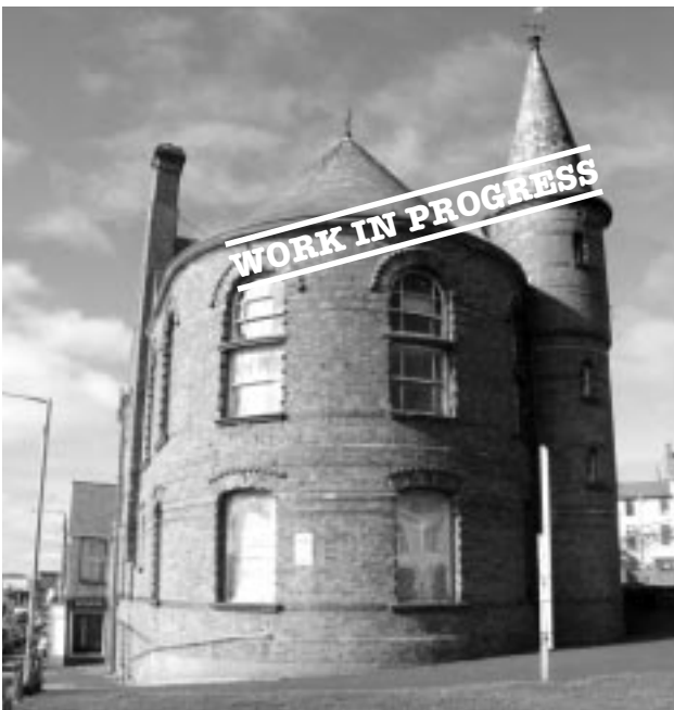
Portrush Town Hall Hearth is currently on site with the restoration and reuse of this important listed building, which appeared in BAR Vol. 2, p. 13. Upon completion it will become a community facility, in association with Coleraine Borough Council.
