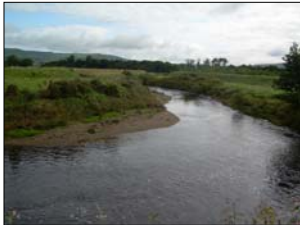
River Roe Flood Banks Limavady
