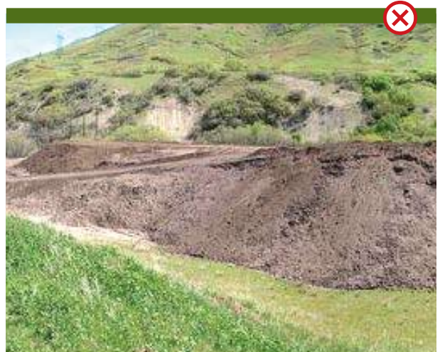
Stockpiling on third party land
