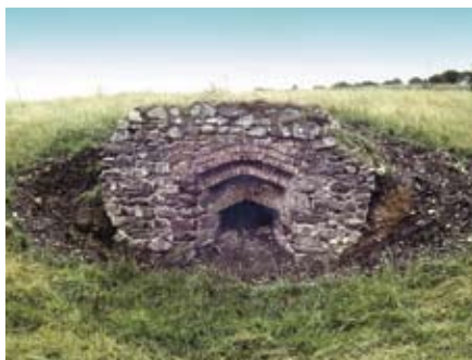
A small farm lime kiln surviving in a good state of repair
