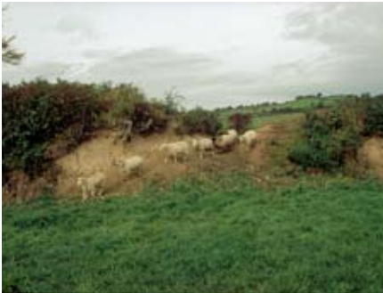
Erosion damage on the bank of a rath at Drumilly, Co. Armagh
