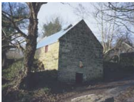
Mullycovet mill after repairs, Co. Fermanagh
