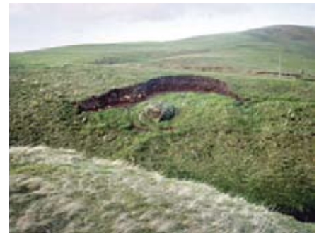
Sheep erosion on the bank of an earthwork prior to repair at Linford, Co. Antrim
