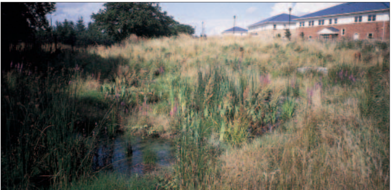
This wetland serves an industrial estate in Livingston. It acts as both a water treatment facility and provides wildlife interest.
