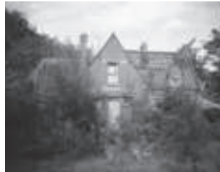
Ormeau Park House, Belfast (before restoration)
