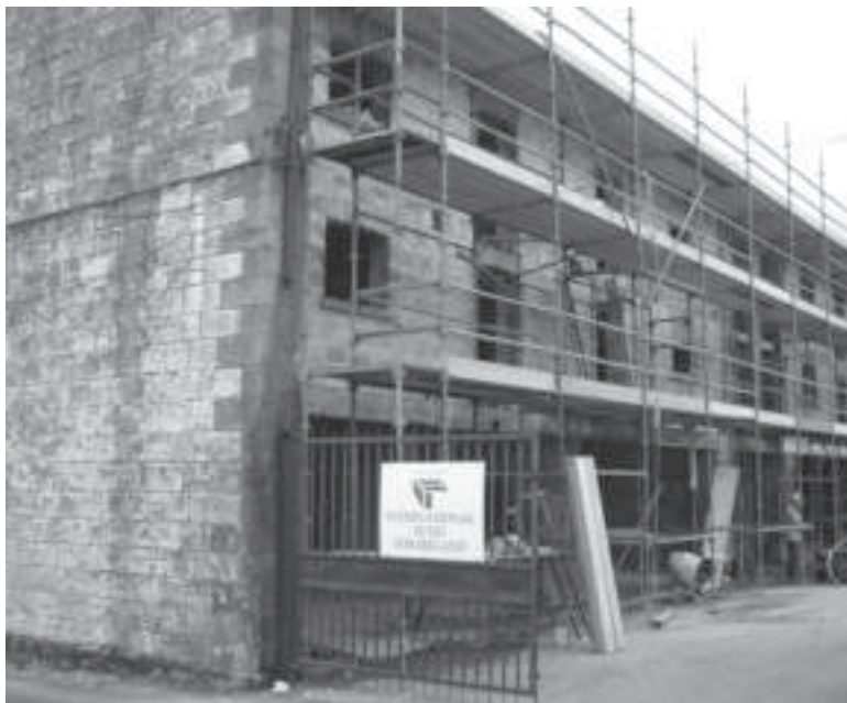
Corn Stores, Market Street, Moneymore (during restoration)
