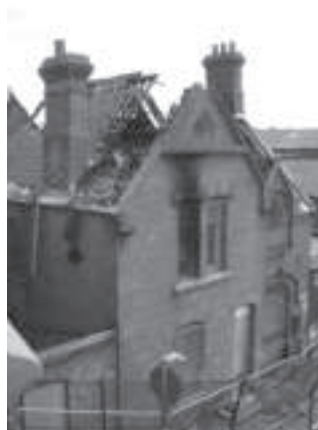
Fire Station, Hawkin Street, Derry (before restoration)
