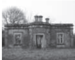
South Gate Lodge, Colebrooke (before restoration)
