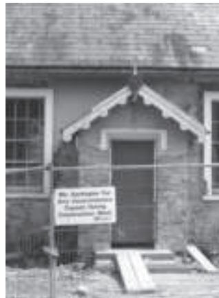
Hollywood Old School, Church Road, (during restoration)
