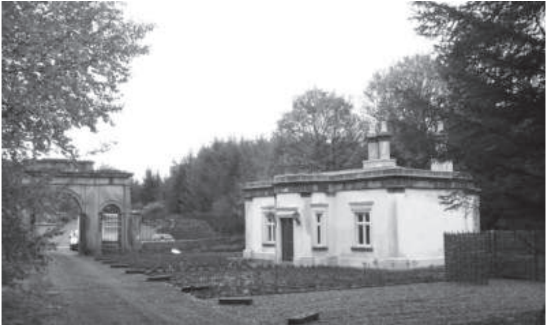
Photo courtesy of Kriterion Conservation Architects
