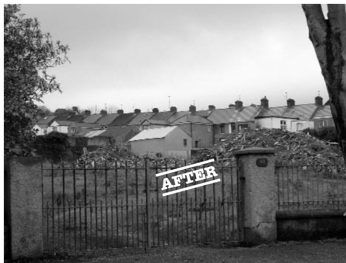
Claremont Lodge, Northland Road, Derry Unlisted, this mid-19th century lodge was demolished leaving a pile of rubble.
