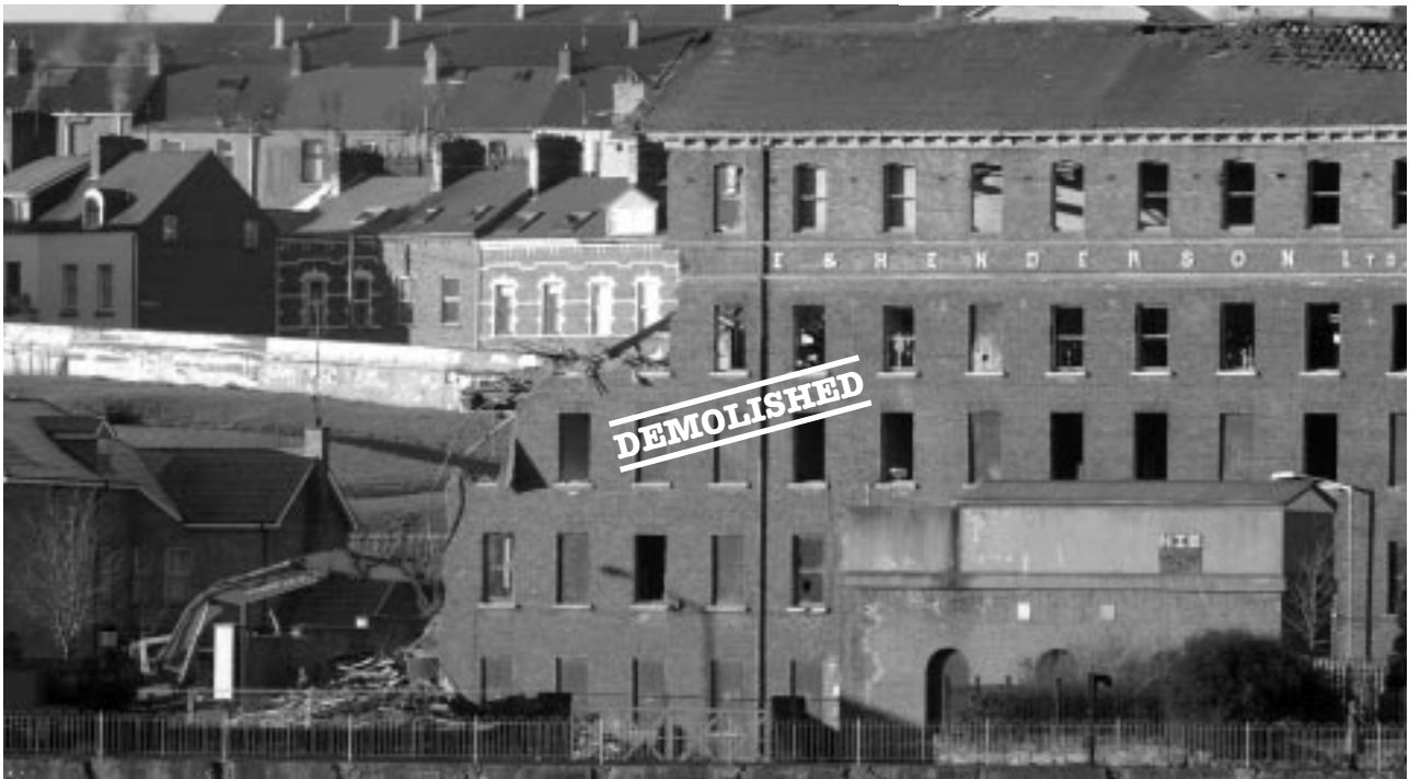
Tillie and Henderson Shirt Factory, Derry Repeatedly fire damaged and demolished without prior authorisation.
