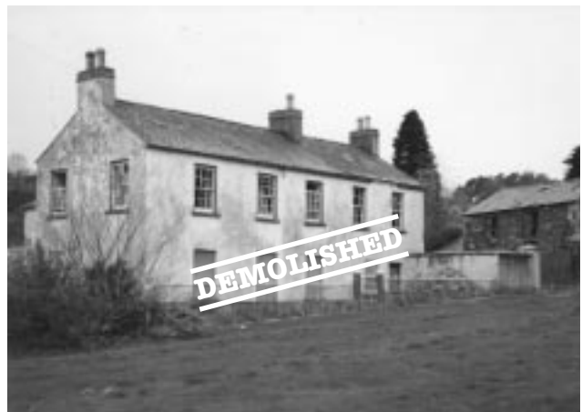
3 Main Street, Markethill Unnecessarily demolished as part of a housing development (BAR Vol. 1, p. 46).
