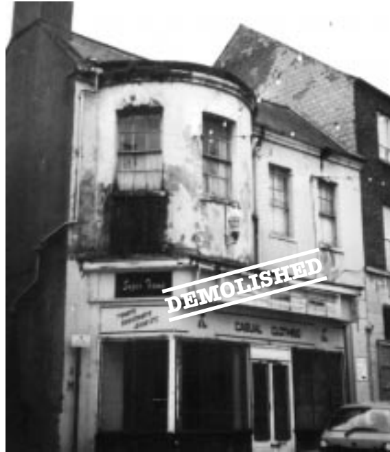
34 English Street, Armagh This unusually bow-fronted Georgian building was demolished without authorisation (BAR Vol. 6, p. 42).
