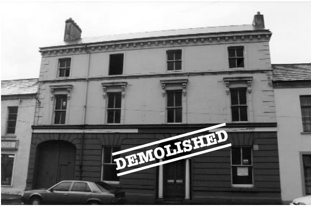
26 Carleton Street, Portadown Demolished and replaced (BAR Vol. 3, p. 30).
