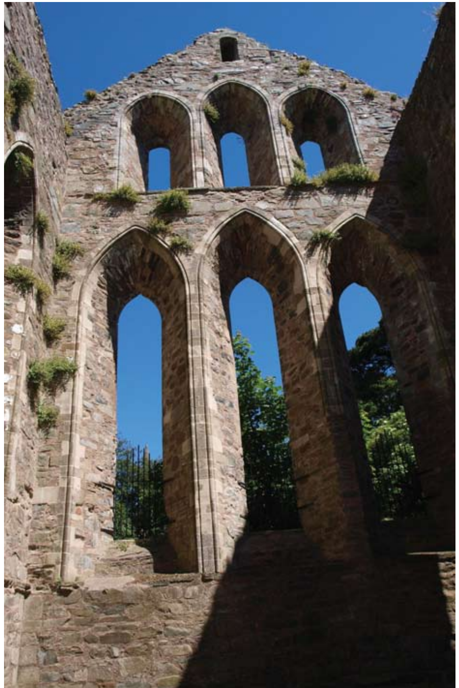
Gothic Lancet Windows on East Wall
