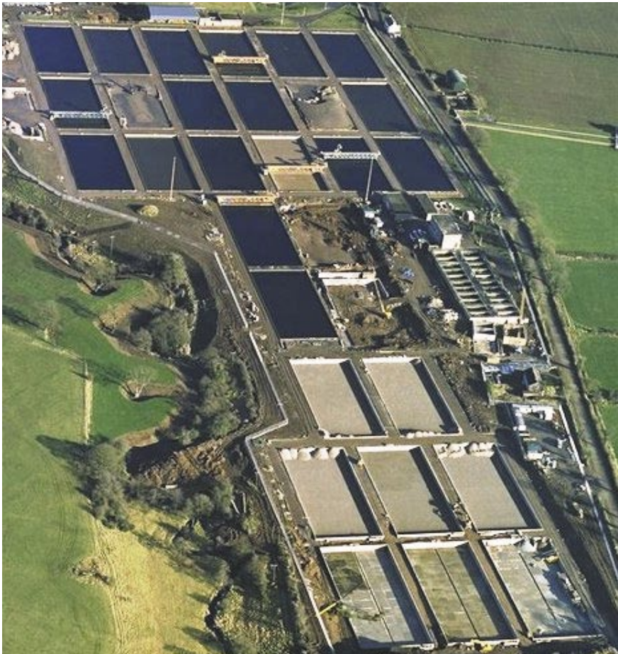
Figure 2: Dunore Point Water Treatment Works
