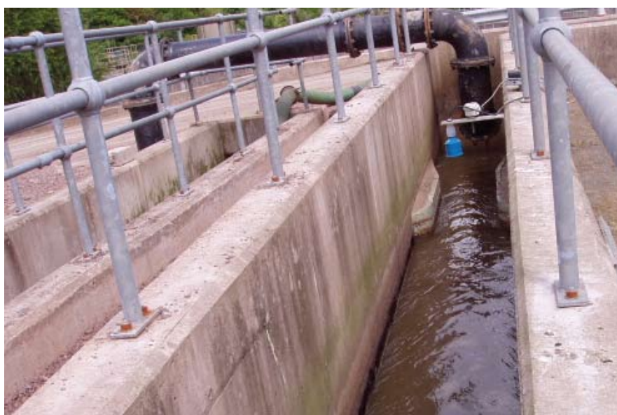
Figure 5: Moygashel Inlet Channel and Flume
