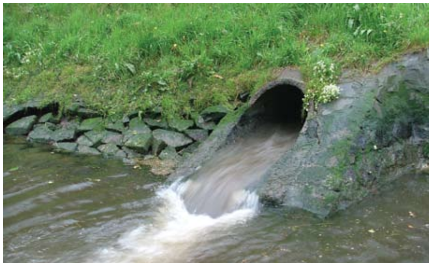
Figure 2. Governors Bridge CSO
