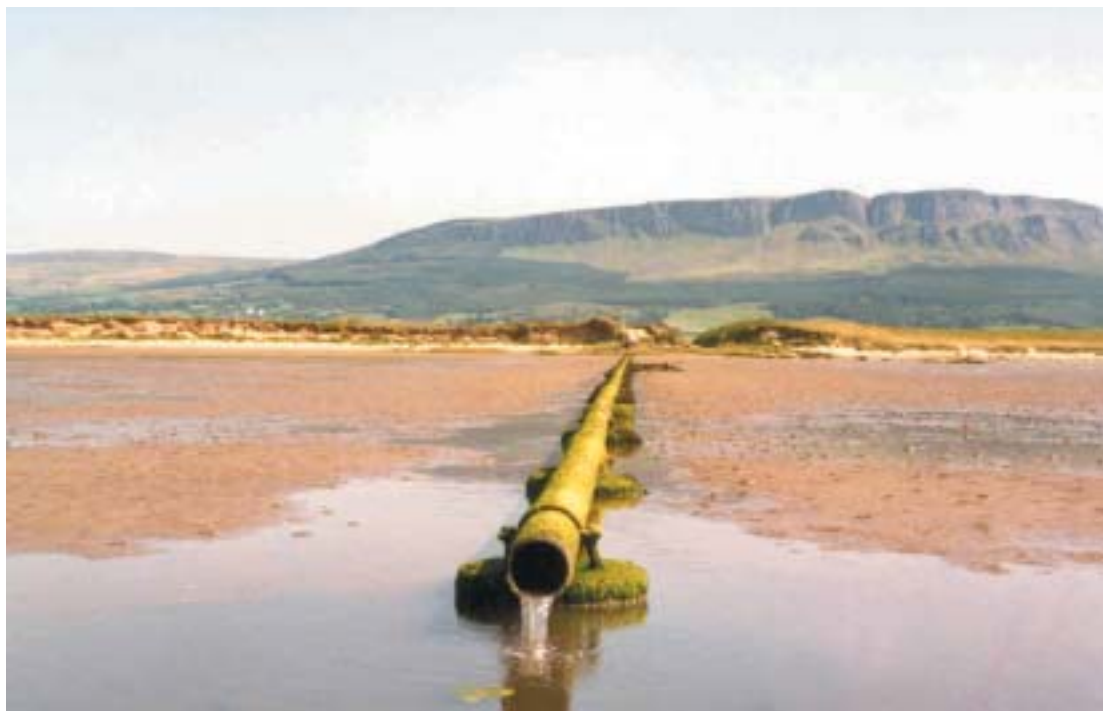
Drumavalley WWTW Outfall
