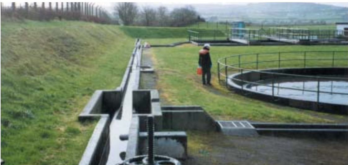
EHS Water Quality Inspector sampling at Castlederg WWTW
