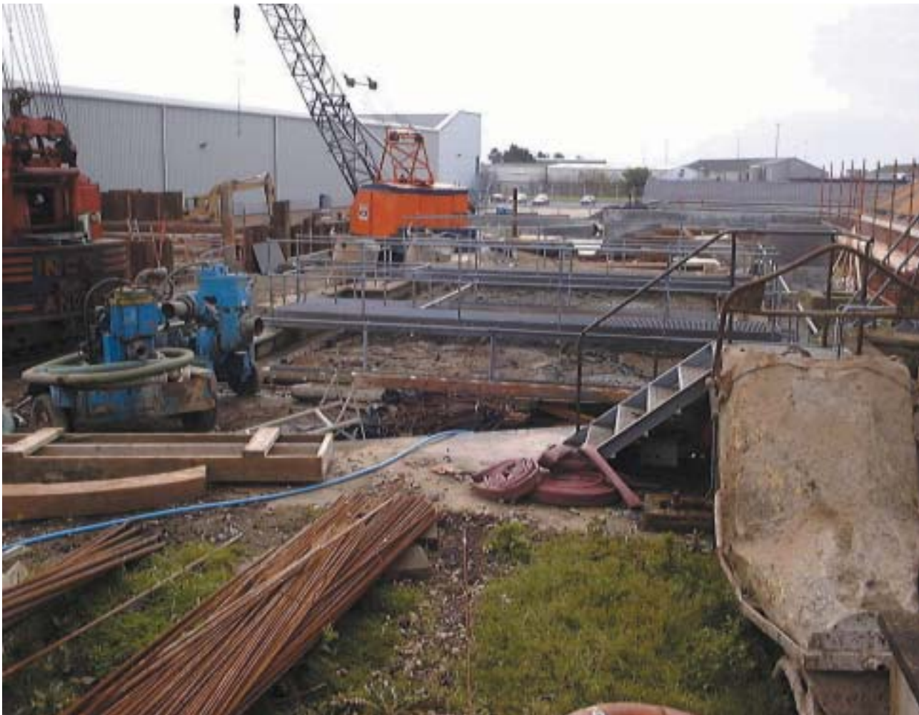
Construction of the new Kilkeel WWTW
