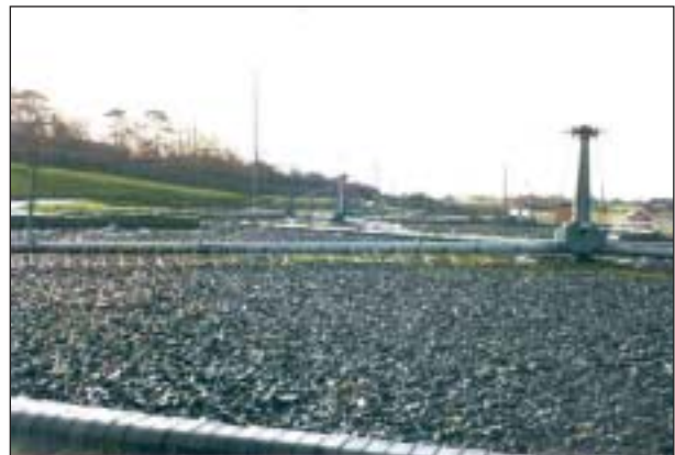
The filter beds at Ballymena WWTW
