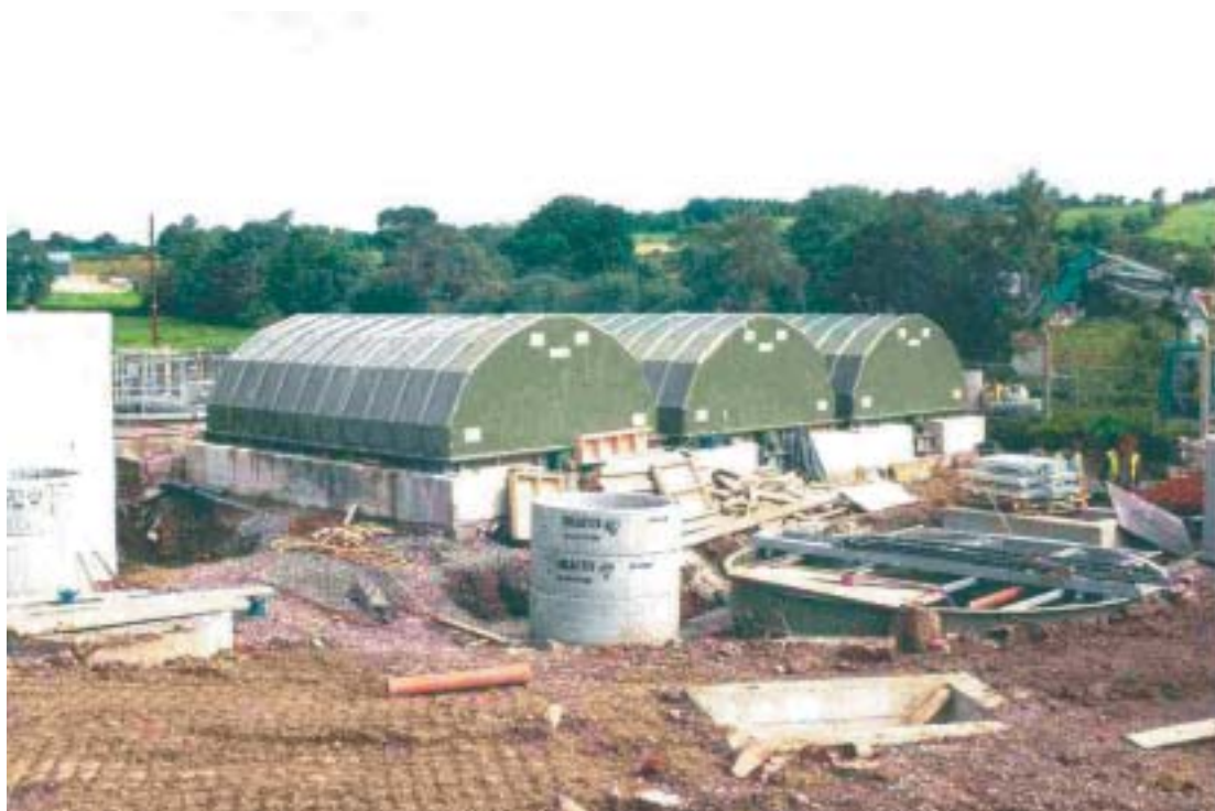
Construction of the new WWTW at Derrygonnelly
