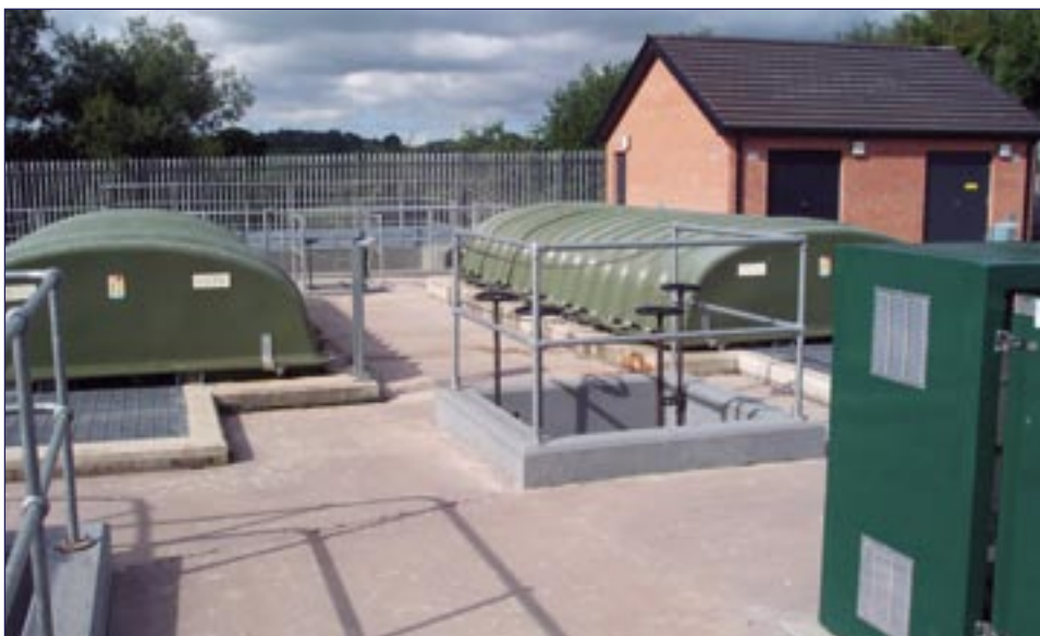
Figure 3: Rotating Biological Contactor (RBC) at Killeen
