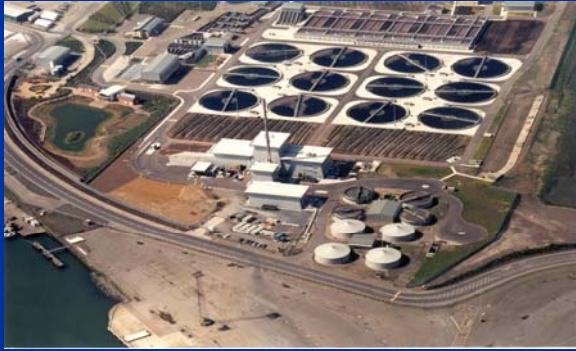
Belfast WwTW - Duncrue St Activated Sludge Plant for 320K PE
