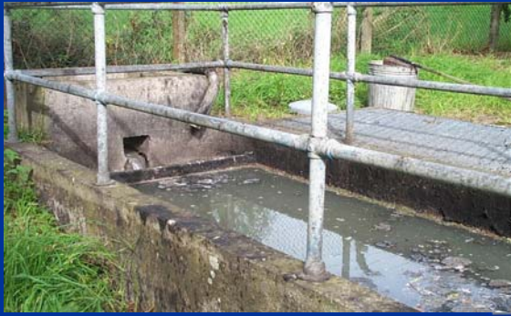
Kinawley WwTW Primary Tank for c100 PE
