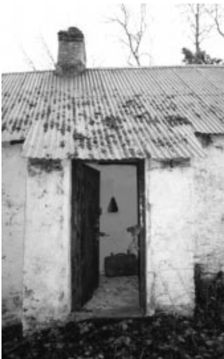
Drumconwell Cottage porch
