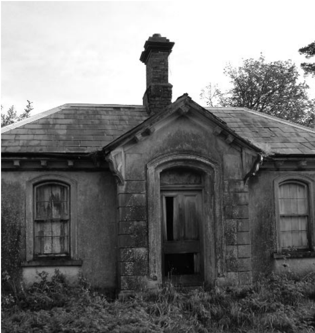
Aghnahoe Lodge before restoration
