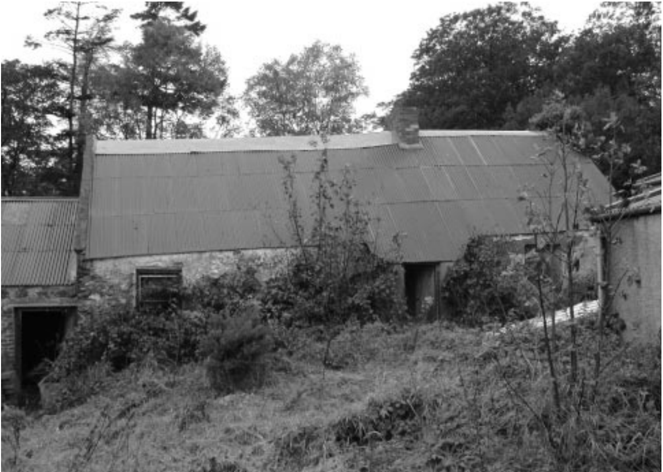
Kilmacrew Road before renovation work
