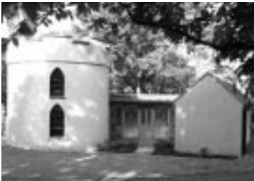
...and after restoration
