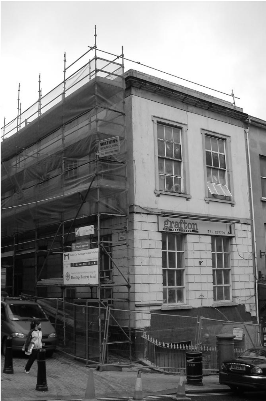
Work underway at 14 Shipquay Street, Derry
