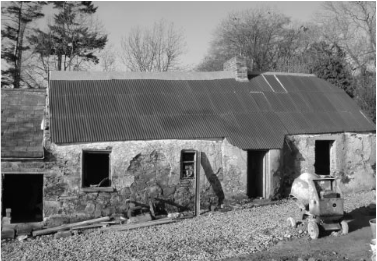
Kilmacrew Road during ongoing renovation work
