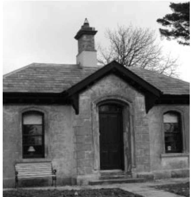
Aghnahoe Lodge after restoration
