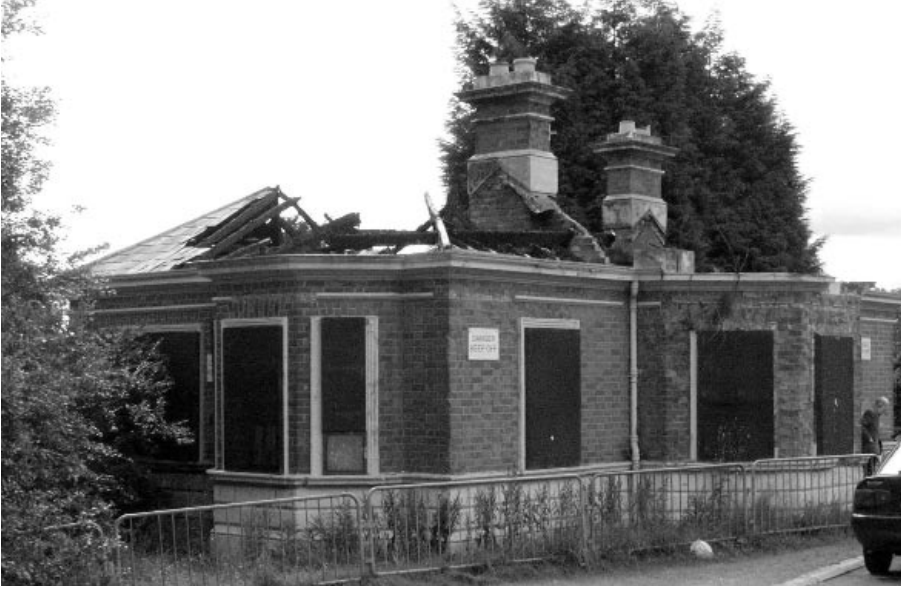
One of the lodges to Wallace Park before restoration
