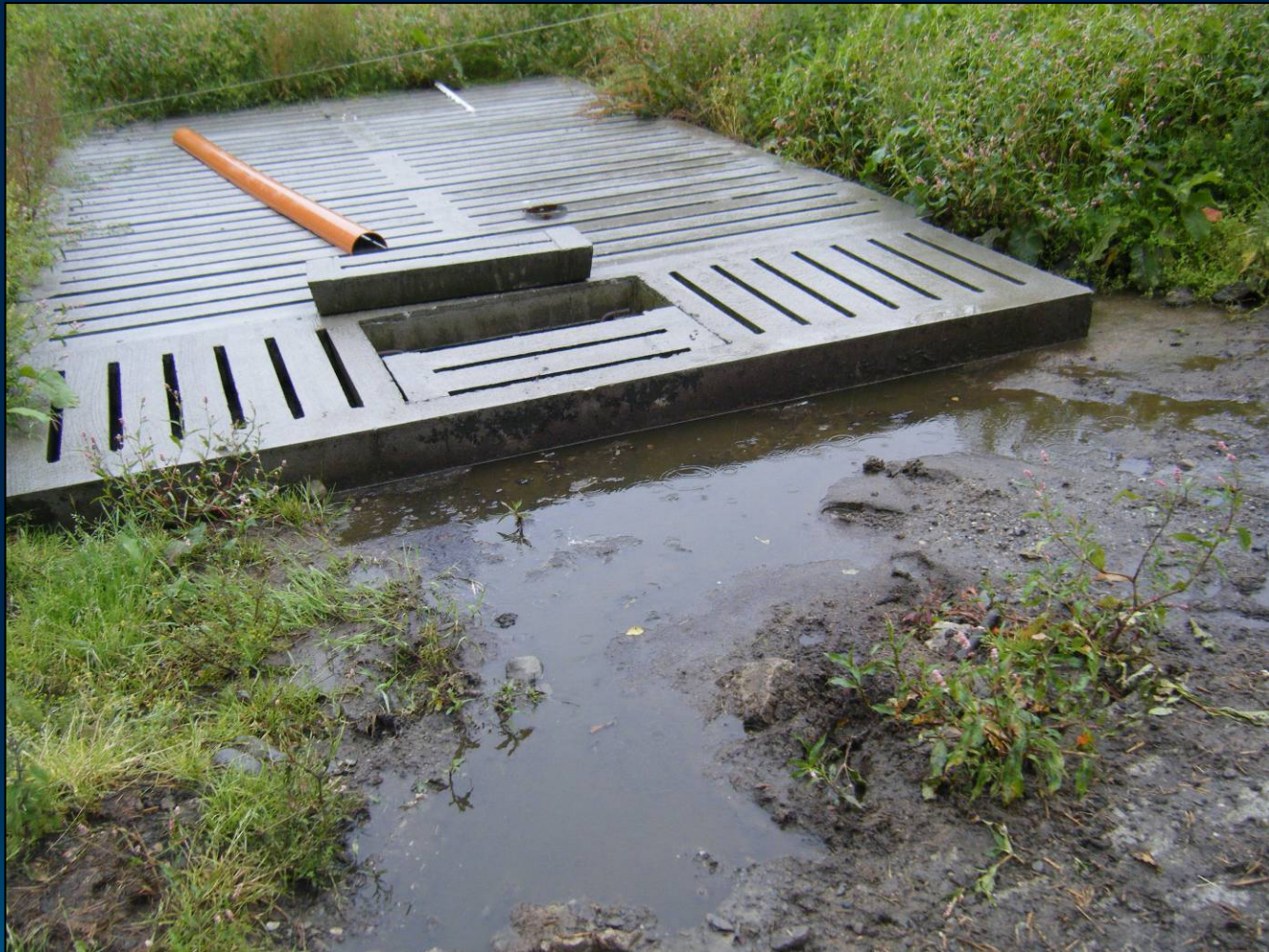
Overflowing dirty water tank
