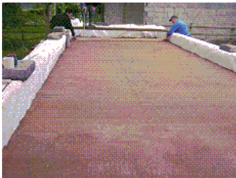
Compact Vertical Flow Reed Bed under construction in Ballynure Co Antrim(NIRBC)
