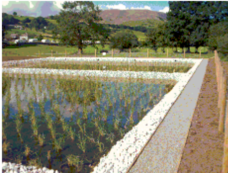
Horizontal Flow Reed Bed
