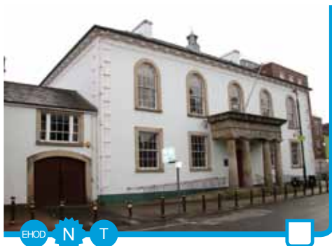
Enniskillen Courthouse East Bridge Street, Enniskillen, BT47 7BP
